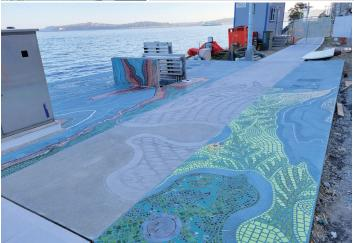
"BILCO hatches were submitted by contractor and met the design requirements," said Avery Reger, P.E., of SPU. "There were limited manufacturers that could produce a hatch with an inlay pan for the concrete and tile artwork that was to be installed. Being able to extend the artwork on to the hatches was important for the artist's vision and hides them in plain sight without affecting the accessibility of the station."
